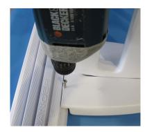
Screw Lower Base of Entrapment Barrier into bottom step of the Inside Portion of the Ladder with (2) #10 x 1-1/4" screws. (This is the side WITHOUT FLIP UP STEPS!)
