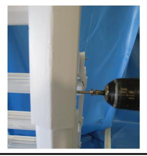
Secure all handrails (AC 01127) to the legs with (4) #10 1-1/4" screws through each of the pre-marked openings.
